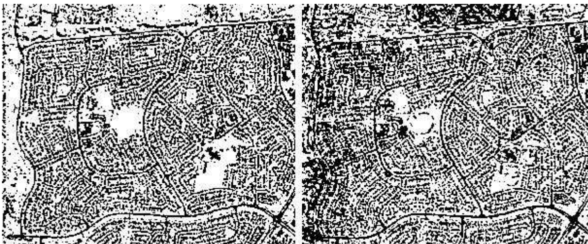
Figure 2: Very high resolution satellite imagery was used to calculate the near infrared reflective index- a measure of surfaces that reflected heat and light- these include roofs, pavements and roads represented by the black pixels. The left side image is 2002 and the right side image is 2006. The western edge of the suburb experienced a 15% increase in built surfaces compared to the unaffected eastern edge. This increase in almost entirely attributed to increased house sizes.
